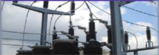
MV Transformer and Switchgear
